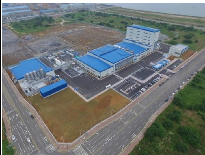
Figure 22: New Gwangyang plant under construction (Oct 2019)
